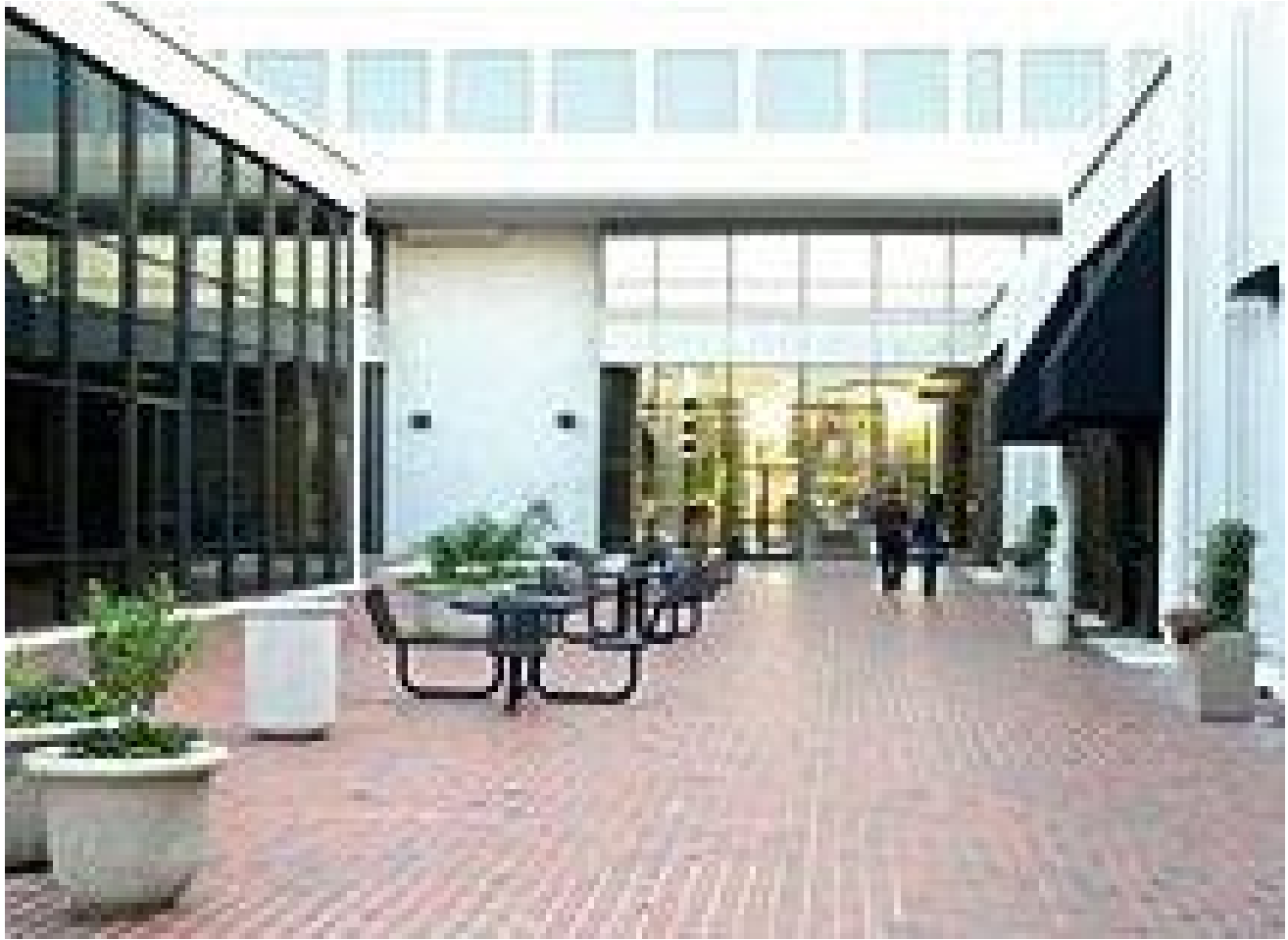
The entrance to Five Branches Institute's new San Jose campus.
